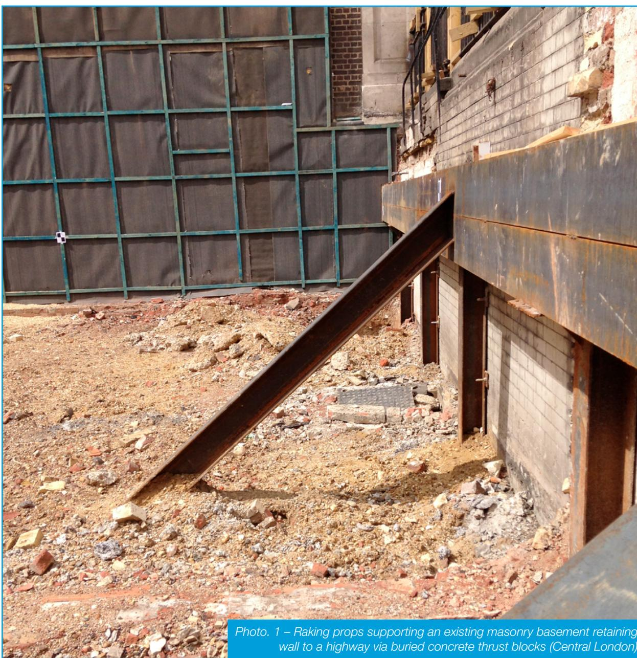
*Photo. 1 – Raking props supporting an existing masonry basement retaining wall to a highway via buried concrete thrust blocks (Central London)*
