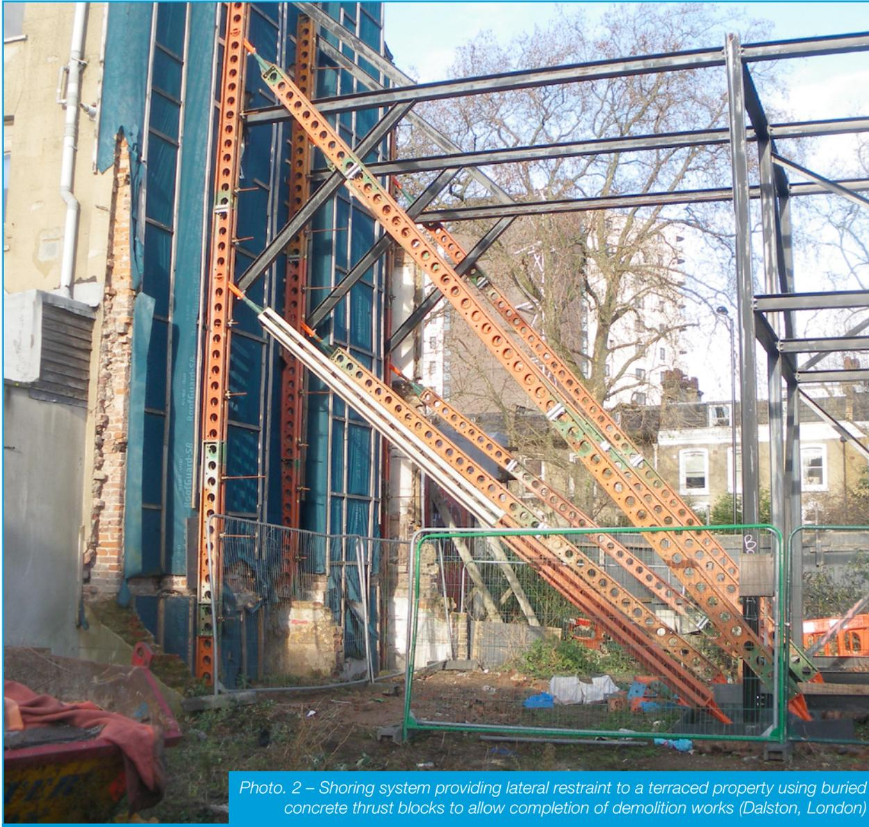
Photo. 2 – Shoring system providing lateral restraint to a terraced property using buried concrete thrust blocks to allow completion of demolition works (Dalston, London)
