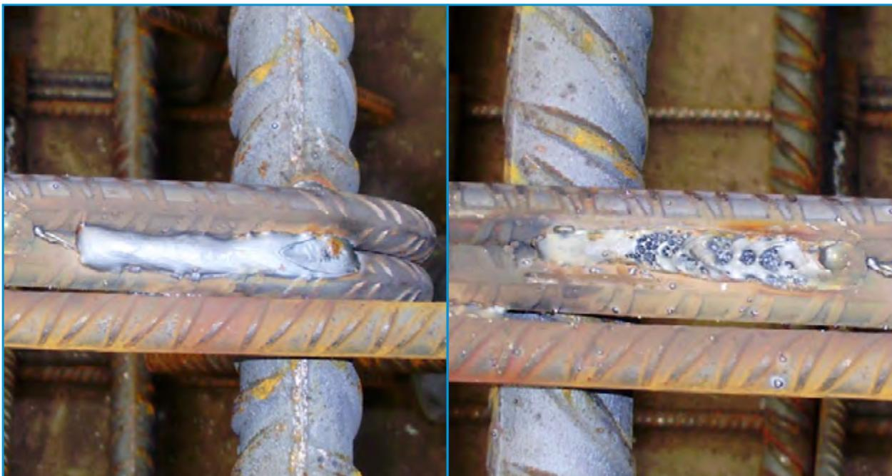
*(a) Insufficient weld to one of the bars so the bars are not effectively joined*
