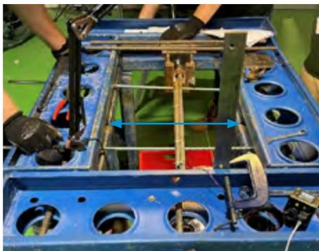
Distance between side soldiers to be kept to a minimum (typically 250mm to 350mm), ensuring there is sufficient space for tying wire.
