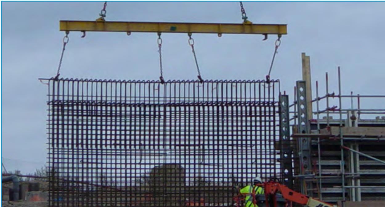
*Insufficient number of drop chains for the size of the cage, inclined drop chains (should be vertical to avoid reactions into the cage), incorrect attachment points and visible deflection of the cage*
