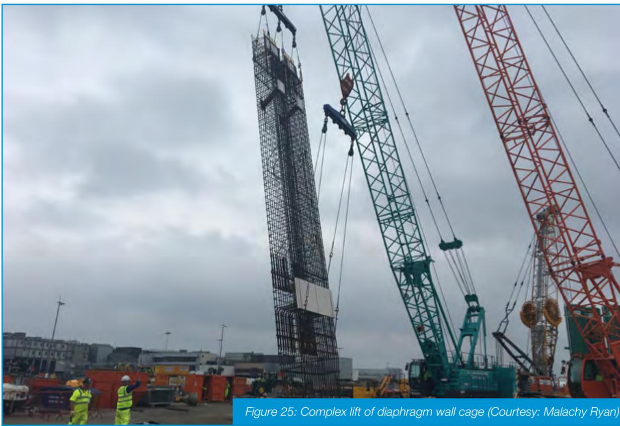
Figure 25: Complex lift of diaphragm wall cage (Courtesy: Malachy Ryan)
