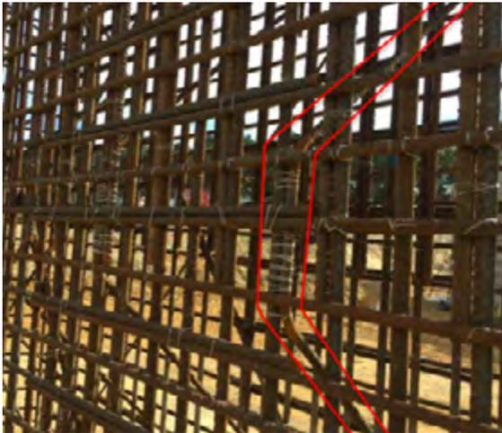
NOTE: Highlighted is a Shape Code 46 (SC46) 'temporary works' stiffening bar, with multiple splice ties connecting opposing faces of the permanent works rebar to provide 'truss action'.
