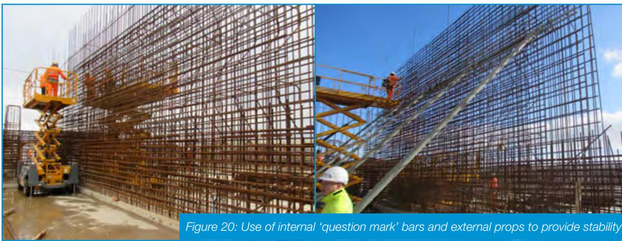
Figure 20: Use of internal 'question mark' bars and external props to provide stability
