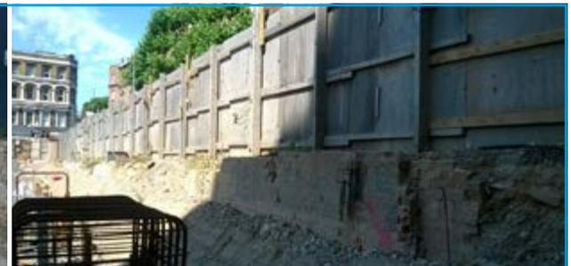
Fig F2 - Example of soil being removed adjacent to hoarding
