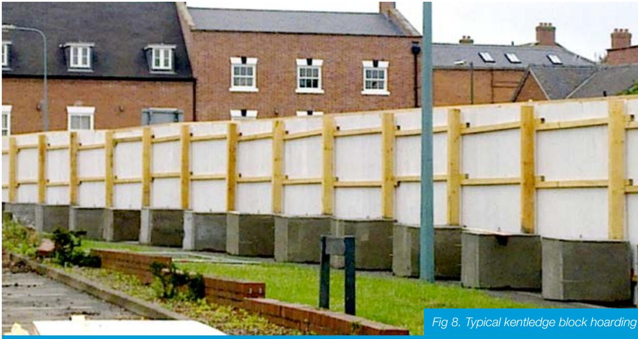
Fig 8. Typical kentledge block hoarding
