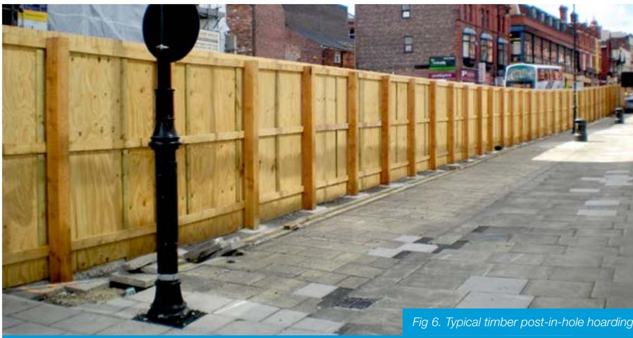
Fig 6. Typical timber post-in-hole hoarding
