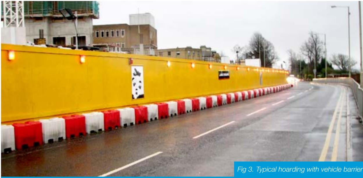
Fig 3. Typical hoarding with vehicle barrier
