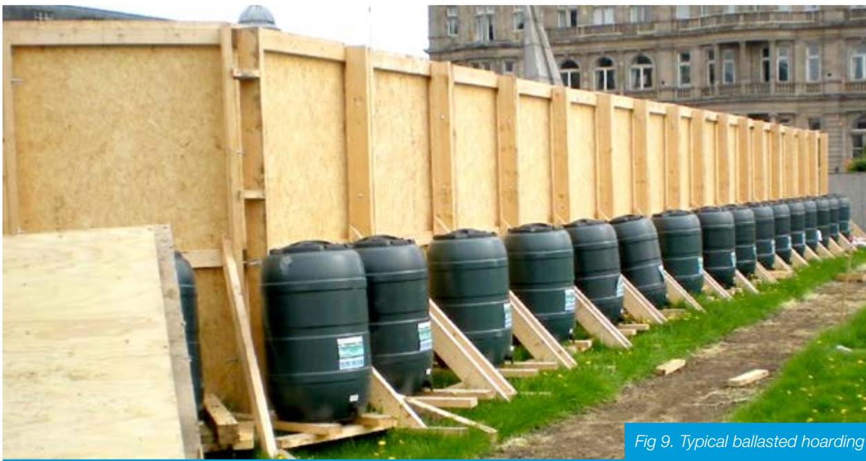
Fig 9. Typical ballasted hoarding
