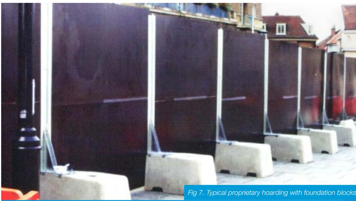
Fig 7. Typical proprietary hoarding with foundation blocks
