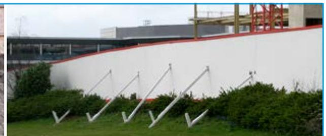
Fig F3 -Example of slope failure leading to a failure of the adjacent hoarding (with emergency remedial measures having been taken)
