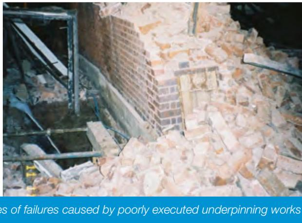
*Photos 3 to 6: Examples of failures caused by poorly executed underpinning works*
