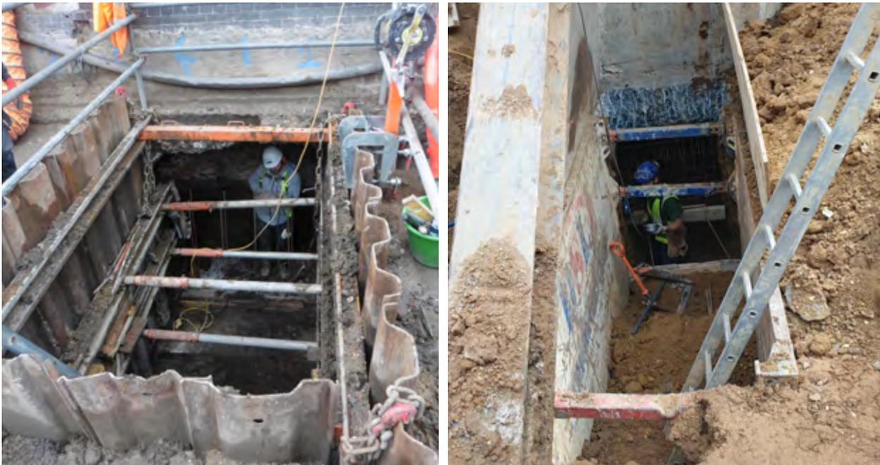
Photos 1 and 2 - Examples of good shoring to access pits for underpinning to external walls
