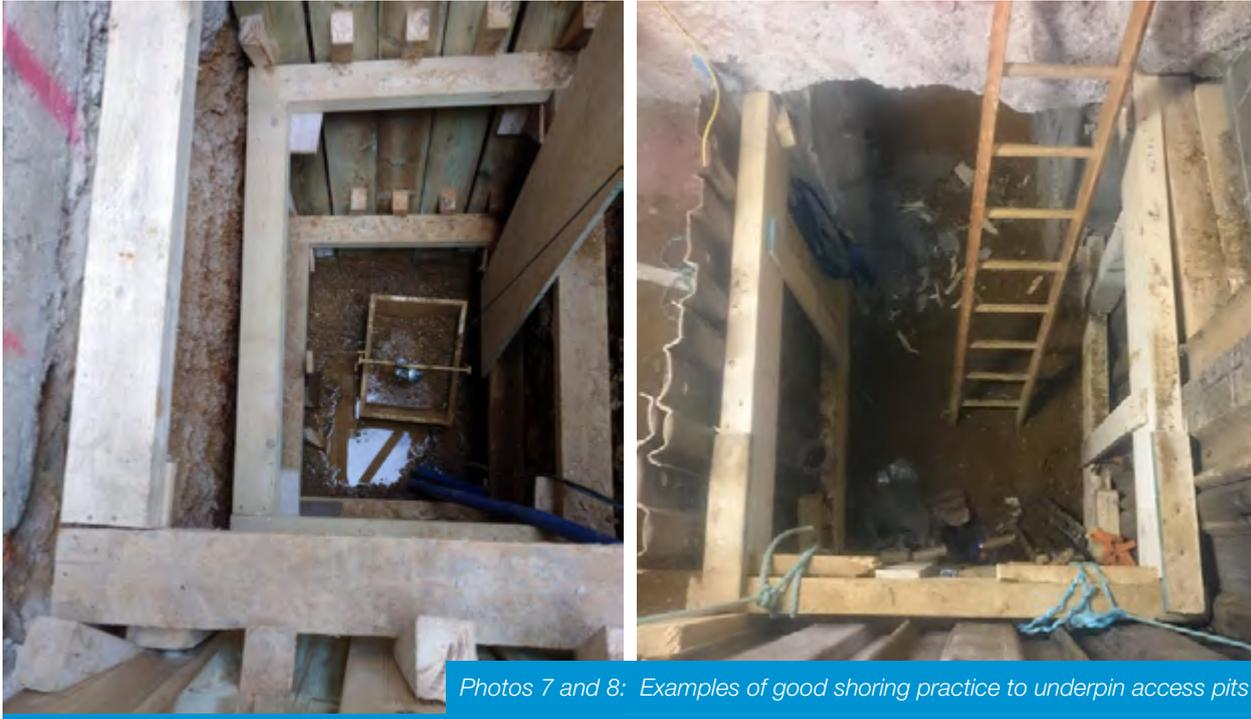
Photos 7 and 8: Examples of good shoring practice to underpin access pits
